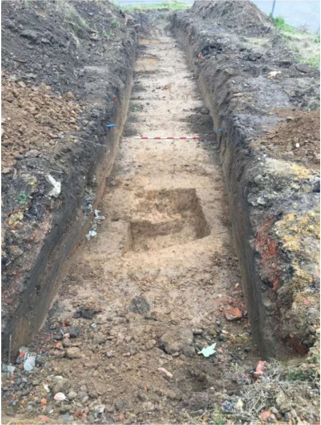
Plate 5. Excavated trench (looking NE)
